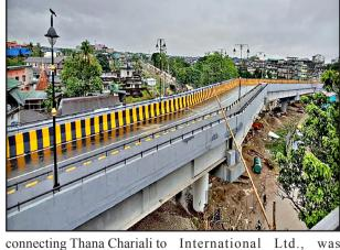
ROB replaces an aging 1965structure to accommodate the growing urban traffic and facilitate Railways' Indian electrification initiative. Designed with a vertical clearance of 6.55 meters, the bridge ensures safe passage of electrified trains while enabling smooth vehicular
